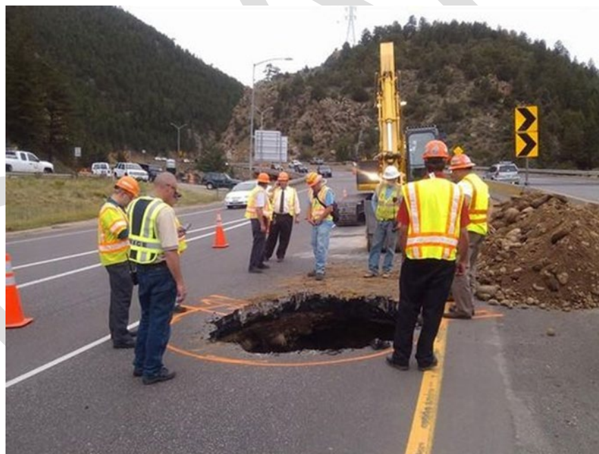
Figure 4-19: Sinkhole on Interstate 70 near Idaho Springs, Colorado, July 19, 2012
